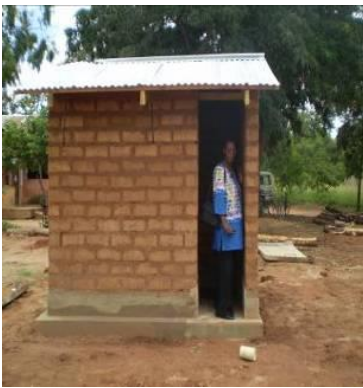
Figure 23: A permanent and durable super structure for privacy and protection from rain, sun, wind etc. Photo's credit: WaterAid
