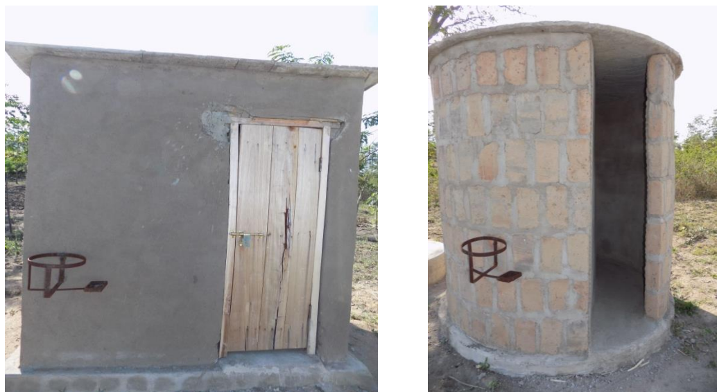
Figure 24: Latrines fitted with hand washing facility stands. Photo's credit: Yolanda Mbatia
