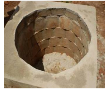
Trapezoidal bricks with dry bonding agent
