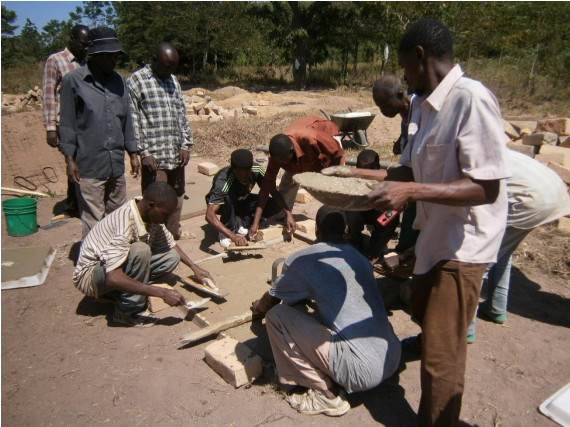
Figure 9: Artisan (TOT) Jeremiah Kataga (with a hat on) instructing artisans on how to make Katoma slab ( a slab which has been innovated by NIMR in collaboration with artisan TOTs and Katoma village artisans). Photo credit: Yolanda Mbatia
