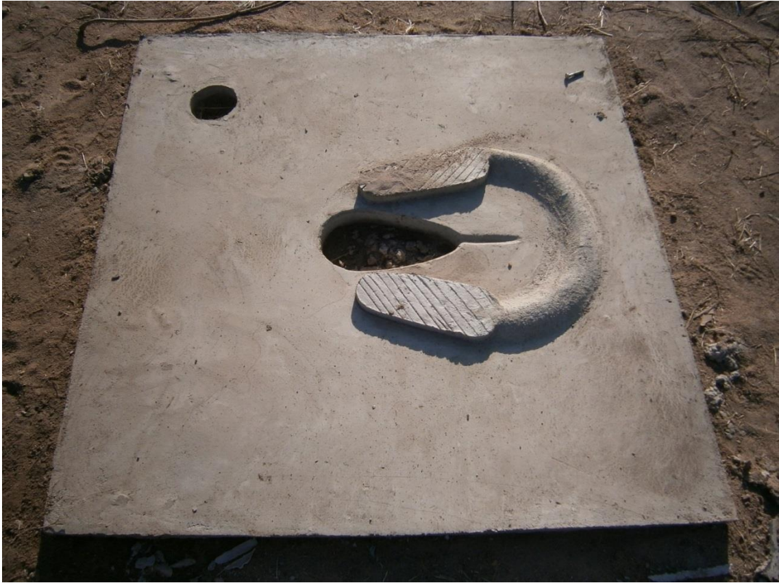
Figure 11: Katoma slab contains urine within a small range and the urine drains back to the drop hole hence less smell and easy cleaning of the latrine. Photo credit: Yolanda Mbatia
