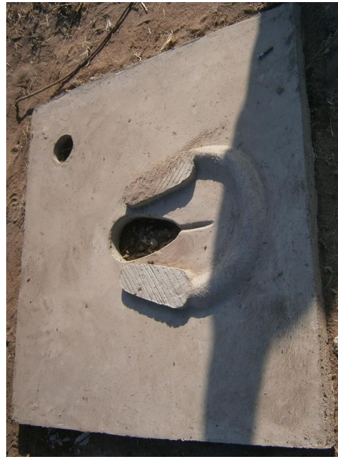
Figure 21: Katoma slab (innovated by NIMR in collaboration with artisan Trainer of Trainers and Katoma village artisans) contains urine within a small range and the urine drains back to the drop hole hence less smell and easy cleaning of the latrine. Photo credit: Yolanda Mbatia
