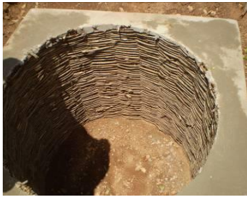
Wattle cage with cement lining
