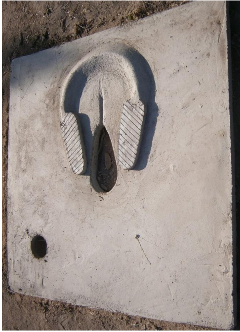
Figure 21: Katoma slab (innovated by NIMR in collaboration with artisan Trainer of Trainers and Katoma village artisans) contains urine within a small range and the urine drains back to the drop hole hence less smell and easy cleaning of the latrine. Photo credit: Yolanda Mbatia
